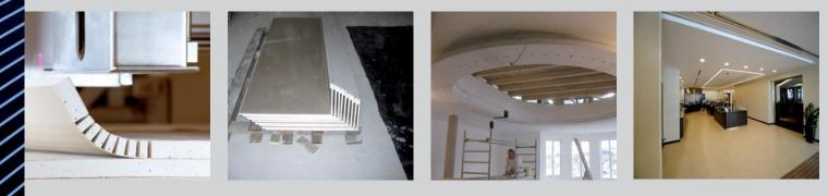
The Supercut XPM from flextos is the first mobile. Self-driving milling machine on the building site, making child's play of corners and edges. There is no more need to set corner protection rails because you can create your own moulds easily without dust directly at the building site straight from the pallet.
